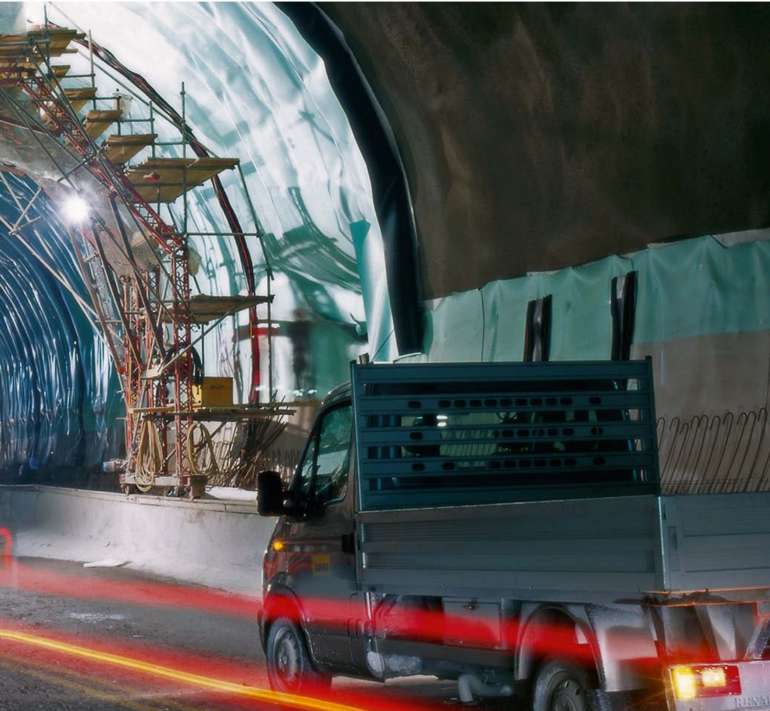
Tunnel Brixlegg, Tirol
